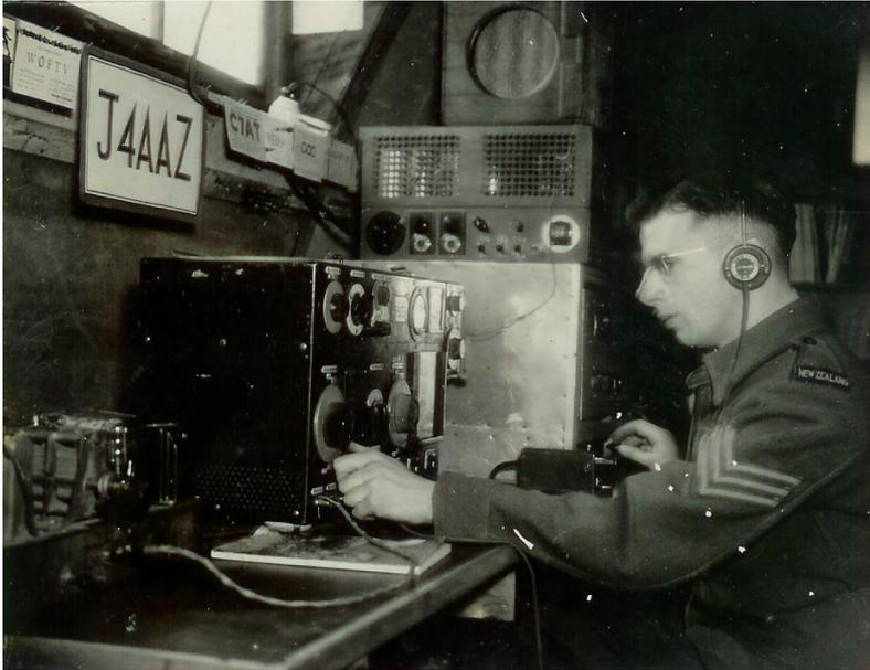
The transmitter was locally built and on the A.M. band (1430 kHz) with a power of about 750 watts. It used a pair of Eimac 250TH's in the final. The antenna was a top-loaded vertical erected by Japanese workmen. It was strung between two 75 feet masts overlooking some rice fields. The modulators were a pair of 100TH's series modulated. The callsign of the station was AKA.A.
