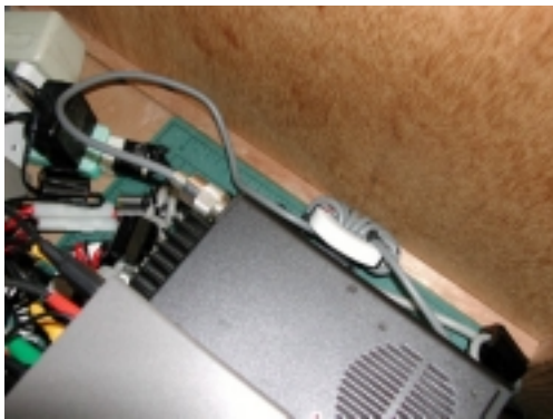
Picture 4: The output feed line of ICOM IC-706mkIIIG is connected to a common-mode filter using an FT-240-43 with 10-turn wound of the 3D-2V feed line.
