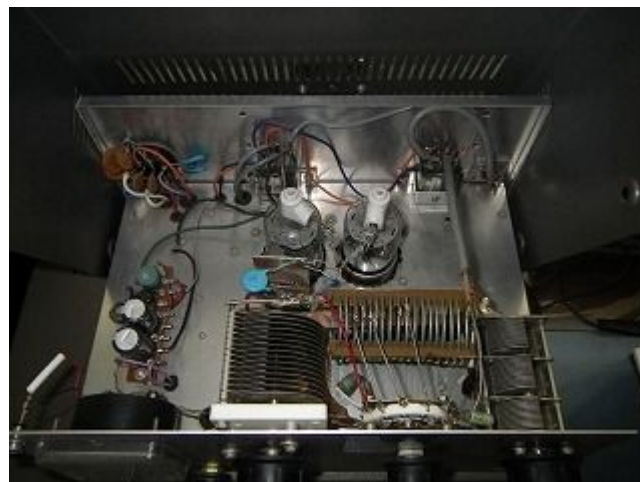
Inside look of the 50-watt linear amplifier using a pair of 6146 tubes.
